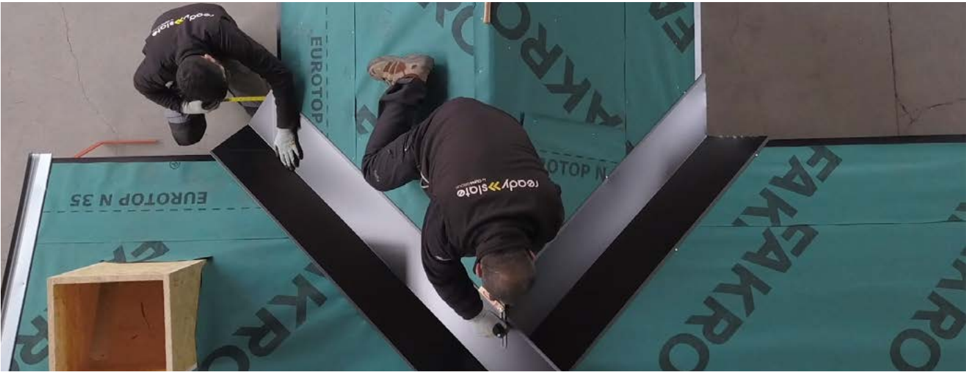
Cut of the READYSLATE® panel to the overlap mark. Continue with the installation of the remaining panels as described before.
